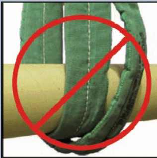
When rigging a basket hitch, DO NOT pull slack out of the hitch with the crane.
